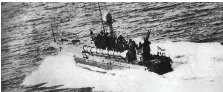
A North Vietnamese P-4 torpedo boat, of the type involved in the Gulf of Tonkin incidents of early August, 1964, is shown underway. The boats, capable of speeds up to 55 miles-per-hour, were equipped with twin 14.7 mm heavy machine guns and two torpedoes. Photo courtesy Bremerton Historic Ships Association.
