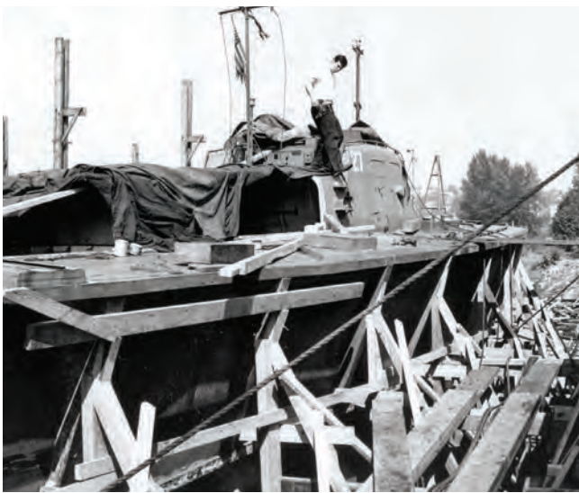
PT-27 is shown undergoing major repair at the Olsen & Winge Marine Works in Ballard during the winter of 1943. The boat had suffered extensive damage in the Aleutian Islands as the result of accidents and operating in harsh weather conditions. Photo courtesy of MOHAI, No. 72.5503.73.
