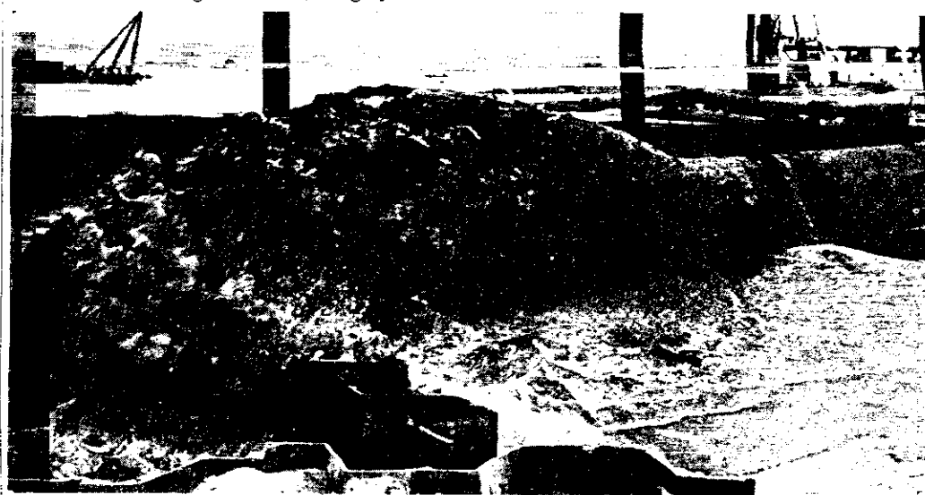
DISCHARGE —Water and sand explode from the dredge discharge pipe into the "fill area." The water is drained off leaving firm sand upon which waterfront facilities will be constructed.
