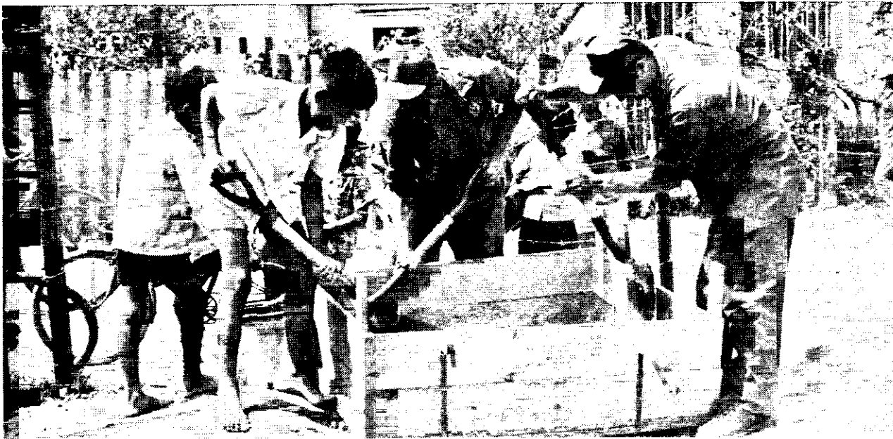
CEMENT MIXER — Firemen J.M. Sumrall and W.K. Carter receive some local assistance as they mix cement for the swimming pool.
