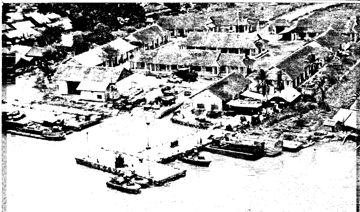
RIVER PATROL BOAT SUPPORT BASE —The Operation Game Warden Base at Vinh Long is a typical NSA Saigon detachment in the Mekong Delta. Two Ammi pontoons joined to form a "T" makeup the main pier.
