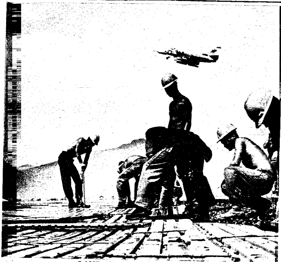
LAND STRIP —The Seabees have laid thousands of yards. (Official U.S. Navy Photo)
