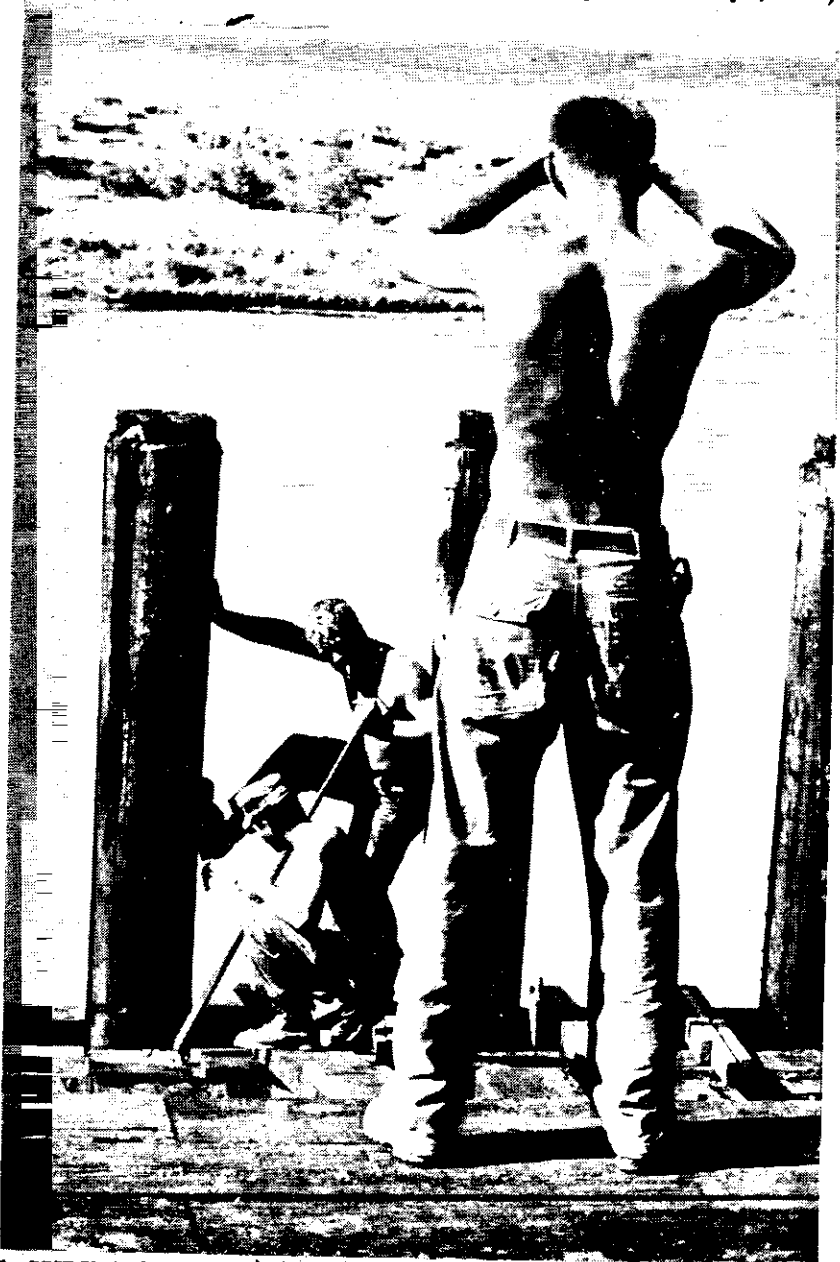
A SURVEYOR lines up one of the 800 piles supporting the Seabee built "Liberty Bridge," in South Vietnam. On far side of the Thu Bon River is the camp of the Marine company which protects the approaching bridge. (Official U.S. Navy Photo)
