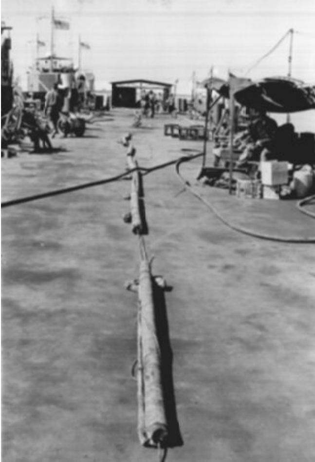
VC Command-detonated mine wire Nha Be
